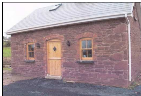
Renovated Kennedy Drummer Cottage at Foilduff
