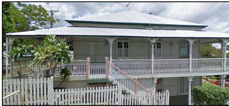
The house Honora built in Brisbane for herself and Martin as it is today
