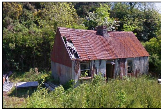
Remains of the Burke cottage at Reafadda
